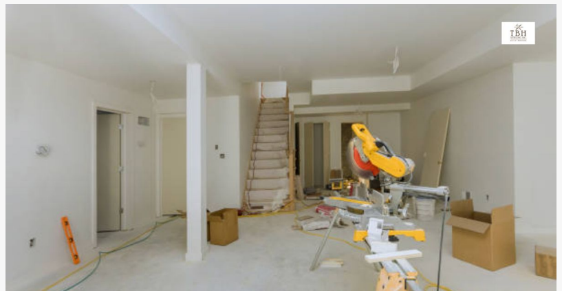
basement remodeling in Seattle
