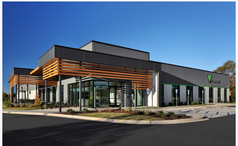
Paxton Access U.S. Headquarters located in Greenville, SC. Designed by MCA Architecture. (Photo courtesy of MPS)
