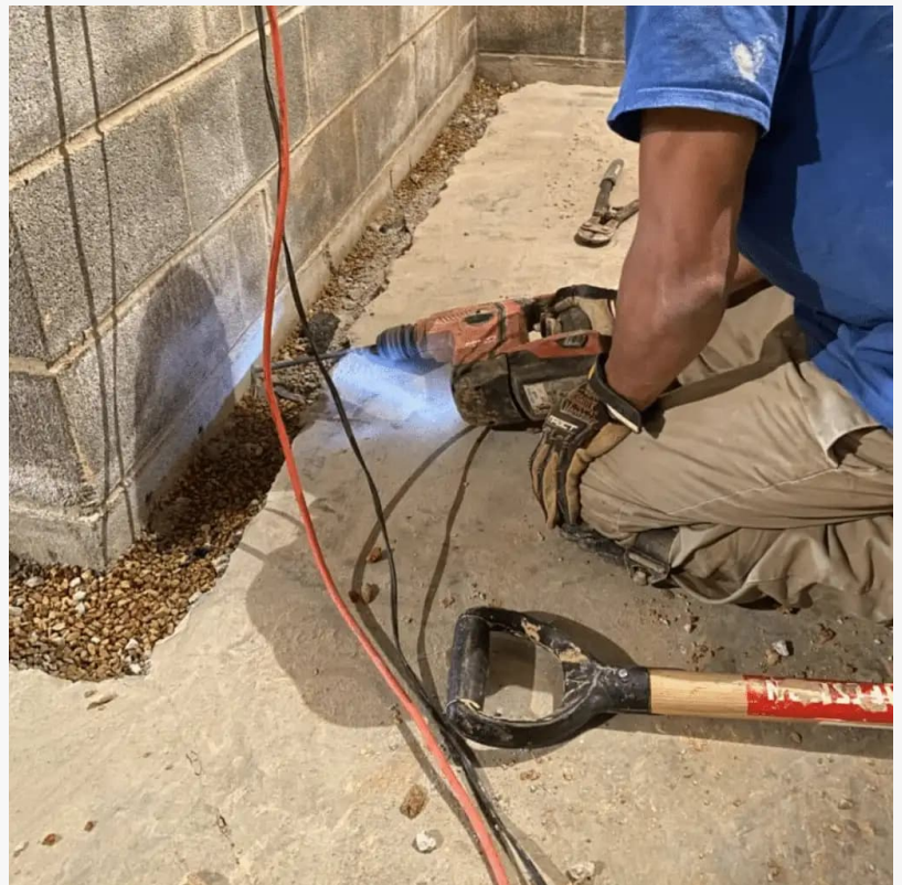
Technician drilling along foundation wall for repair
