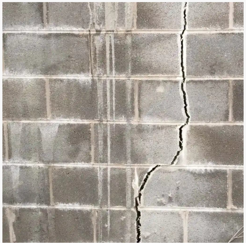
Large vertical crack in foundation wall indicating structural issues
