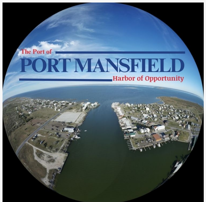
Aerial view of the entrance to the Port of Port Mansfield
