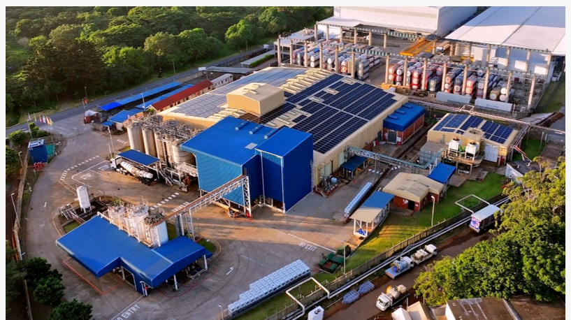
BASF's dispersion-production building at the Durban site, South Africa.
