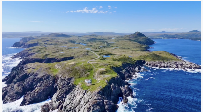
Aerial View of NordSpace's Atlantic Spaceport Complex (ASX) Space Launch Complex (SLC) 02 Under Construction, Newfoundland and Labrador
