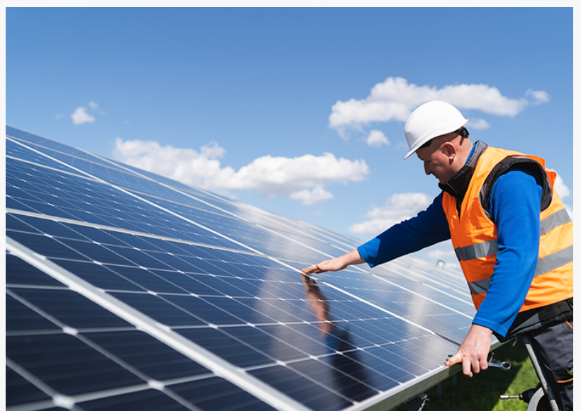
commercial solar energy Garfield
