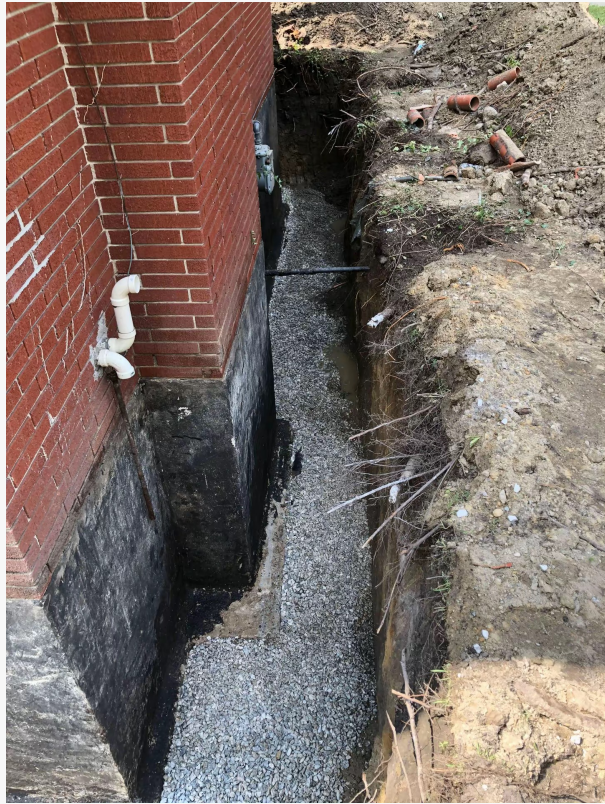
Exterior Basement Waterproofing
