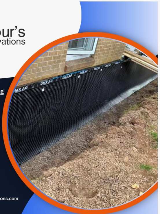
Exterior Basement Waterproofing
