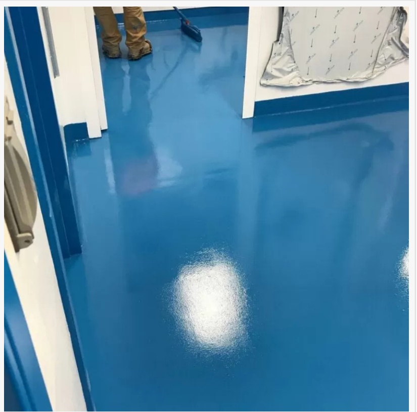
Expert Epoxy Floor Contractor
