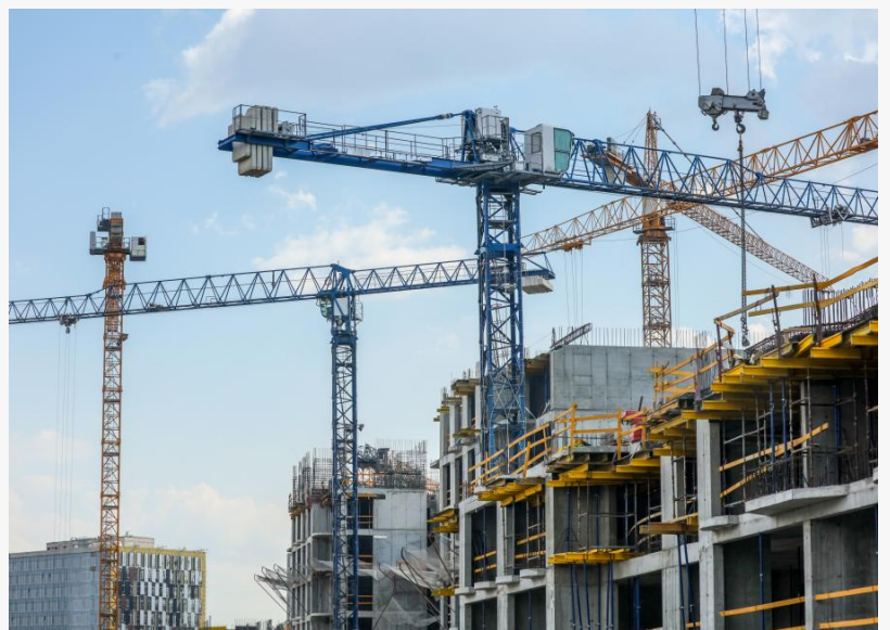
Large-scale construction projects are increasing demand for workforce housing nationwide.
