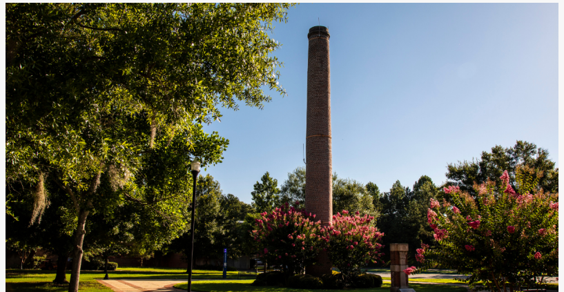
Albany State Chimney
