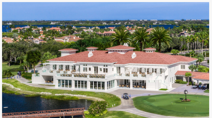
Main Clubhouse Renovation
