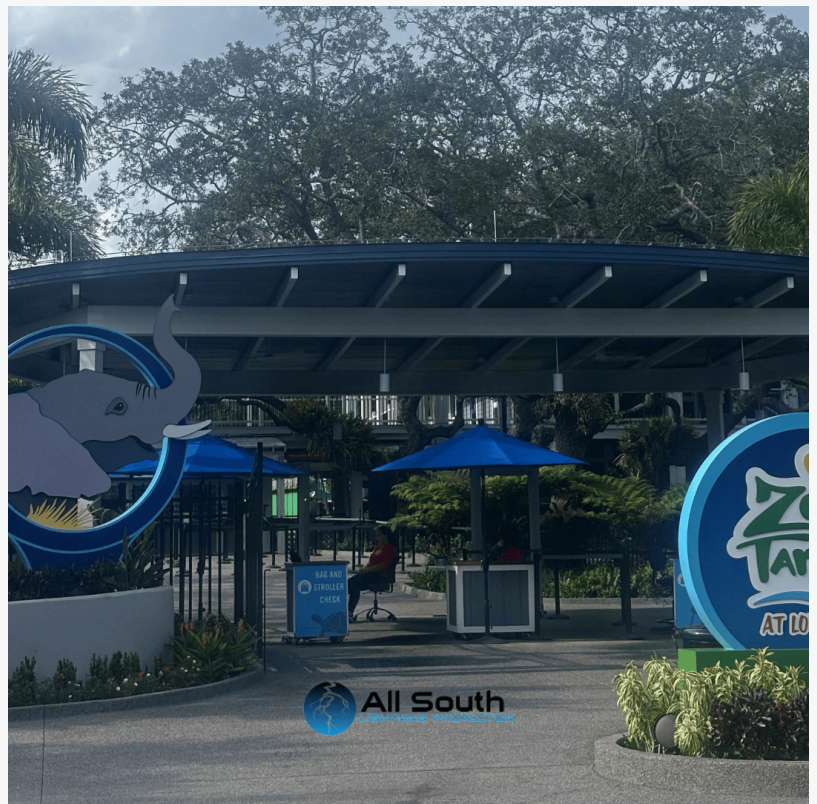
All South Lightning Protection Installation Project Zoo Tampa
