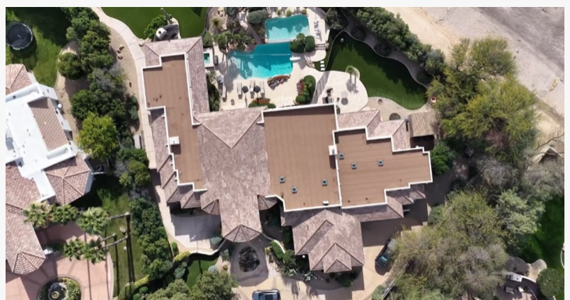
"Old World" Tile Roof System in Phoenix
