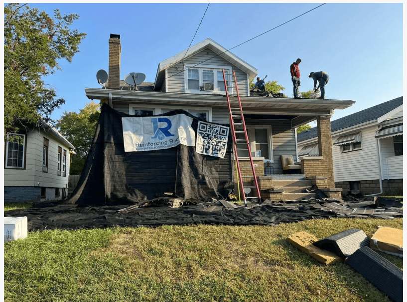
Rainforcing Roofing Experts Performing a Code-Compliant Full Roof Replacement in Peoria
