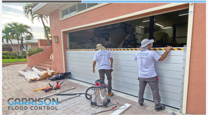
Garrison Flood Control Installation Division
