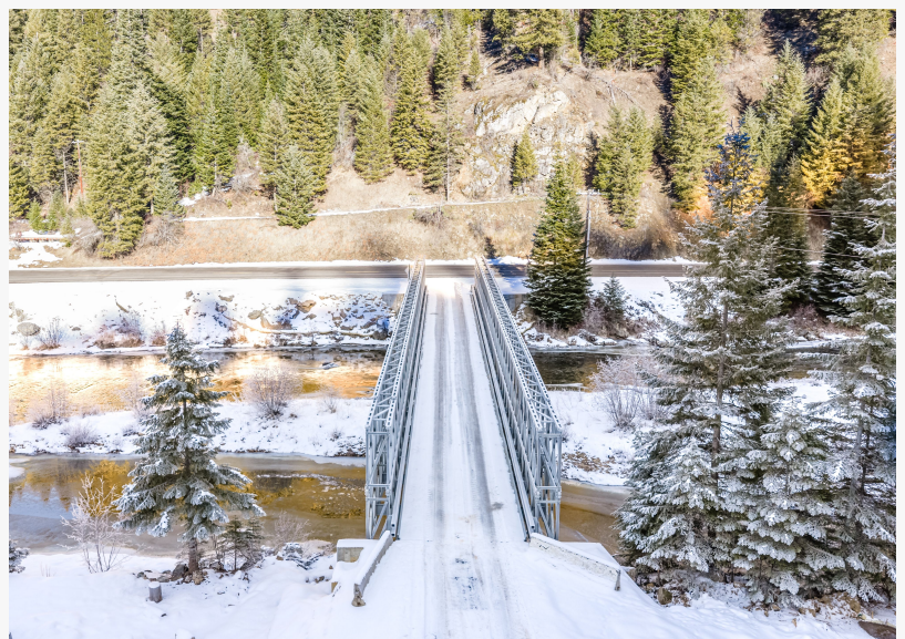
Acrow Permanent Bridge in Golden, Idaho
