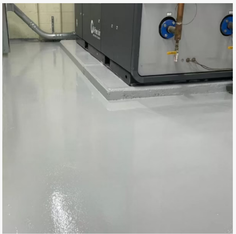
Mechanical Room Floor
