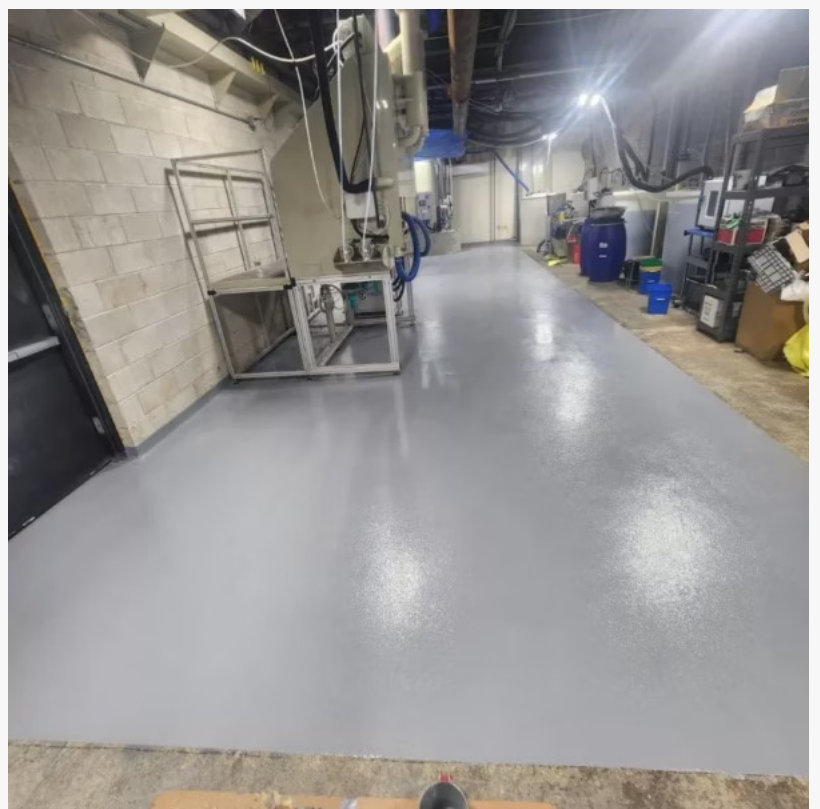
Mechanical Room Flooring
