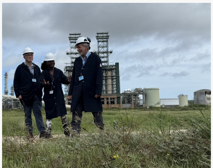
Tom Williams (VP of Operations), Ola Ajala (Principal Engineer), and Kevin Wolf (CEO) surveying the coke dock project site
