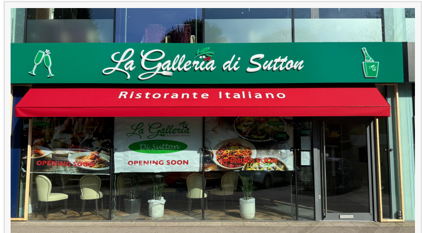
La Galleria di Sutton Work in progress.
