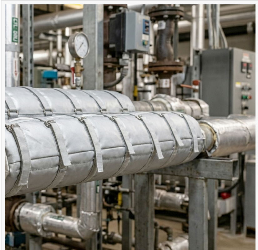
A removable insulation jacket applied on an industrial pipeline, designed to provide thermal insulation, reduce heat loss, and enhance on-site personnel safety in high-temperature environments.
