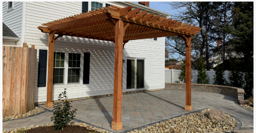
Premium Cedar Pergola Kit Installation by Pergola Depot PRO Contractor
