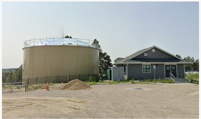
Deer Creek water plant facility
