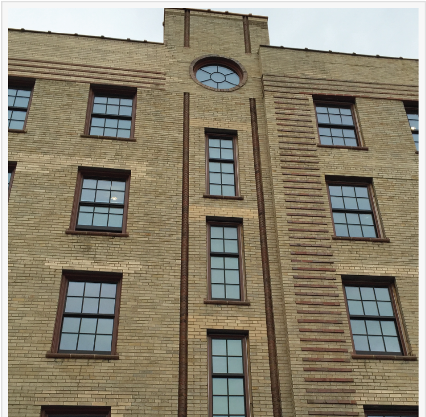
Historical windows renovation works is popular in Europe
