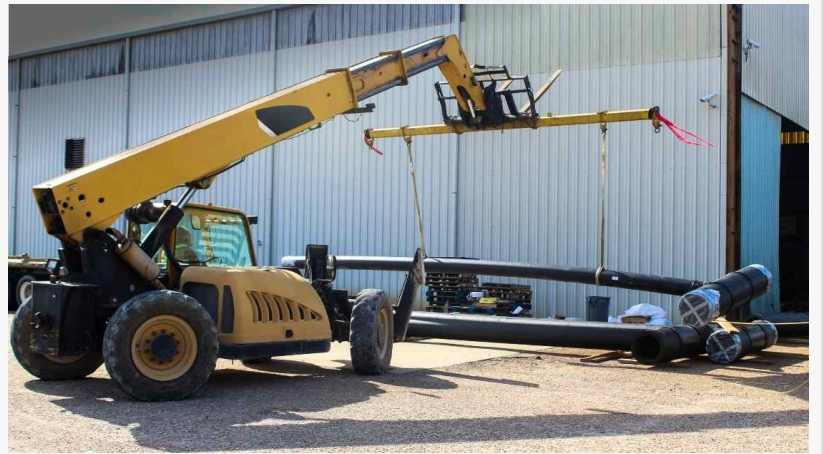
HDPE spool assemblies fabricated, QC-checked & loaded
