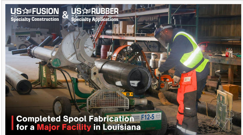
Completed Spool Fabrication for a Major Facility in Louisiana
