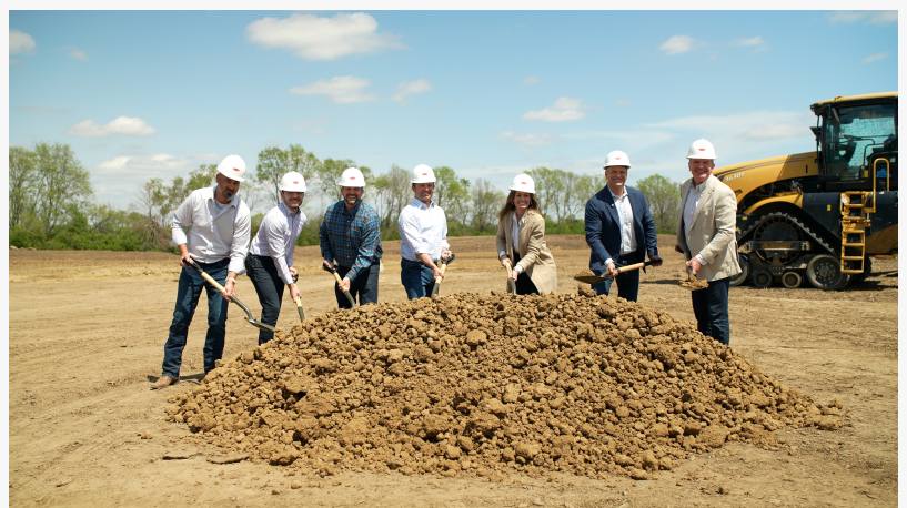
Estridge Homes breaks ground on Millbrook, a 345 acre master planned residential and mixed use community in West Lafayette, Indiana.
