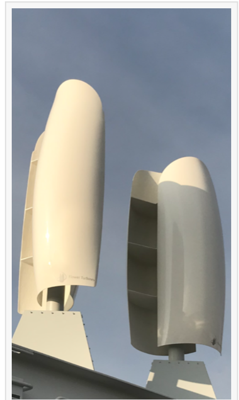
Two Medium Size Wind Tulips Installed
