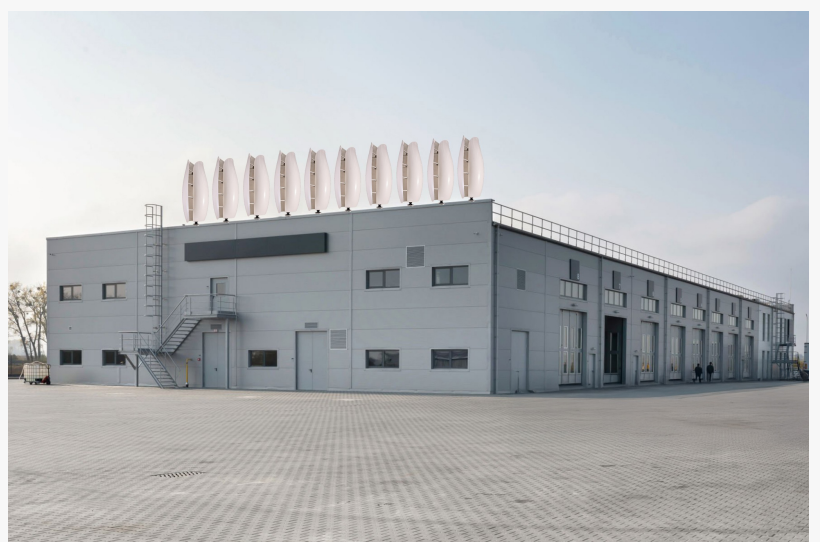
Row of wind turbines on roof
