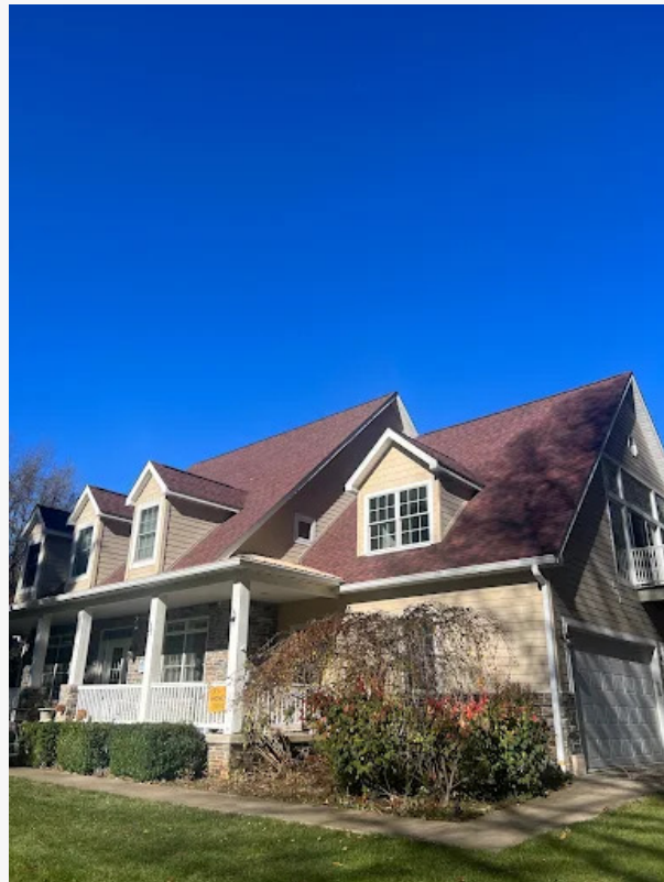
Roof Repair Near Me
