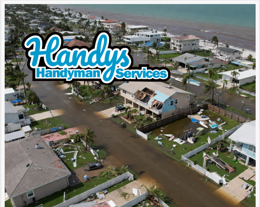
Handys.Now - Sarasota Flood Damage And Repairs
