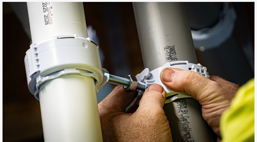
InnoFlue and InnoFlue Lite with OctoClamps being installed by contractor
