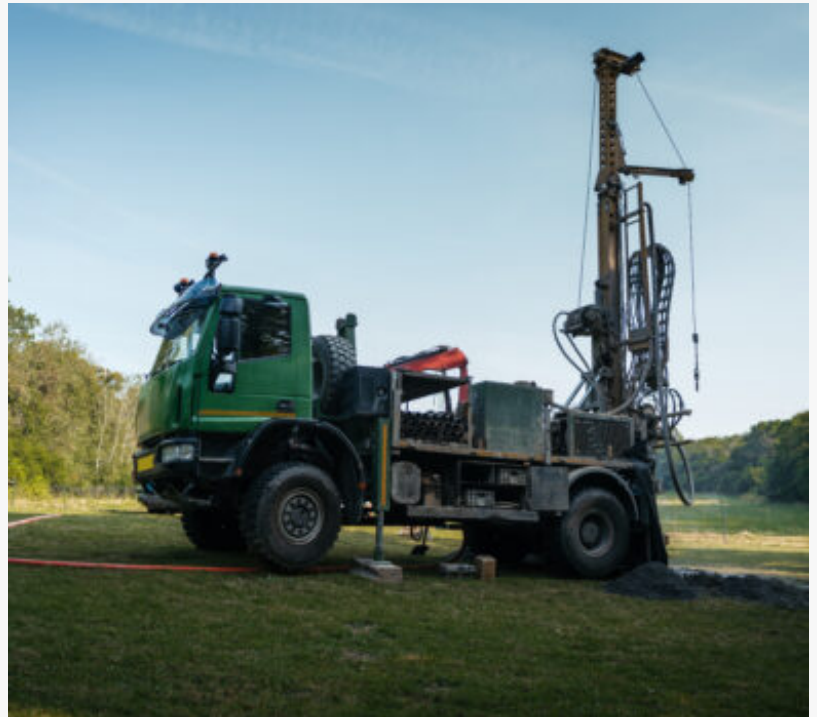
Well Drilling Services in Dover, Delaware
