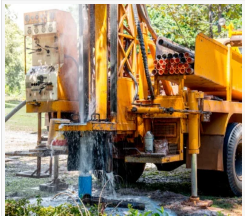
Professional Well Servicing in Delaware
