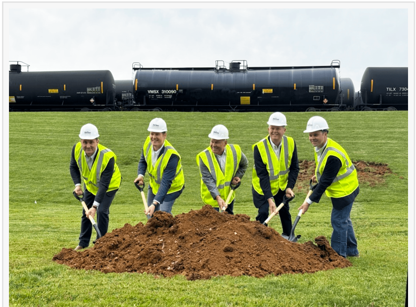
Representatives from Rhoads Energy and community leadership break ground on Rhoads new biofuel center
