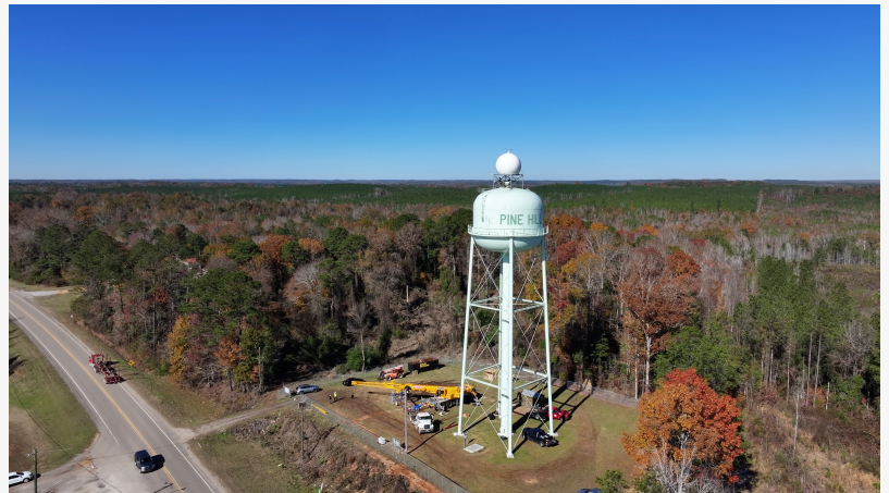
The Climavision radar in Pine Hill, AL covers an area in Southwest Alabama that has lacked coverage for decades
