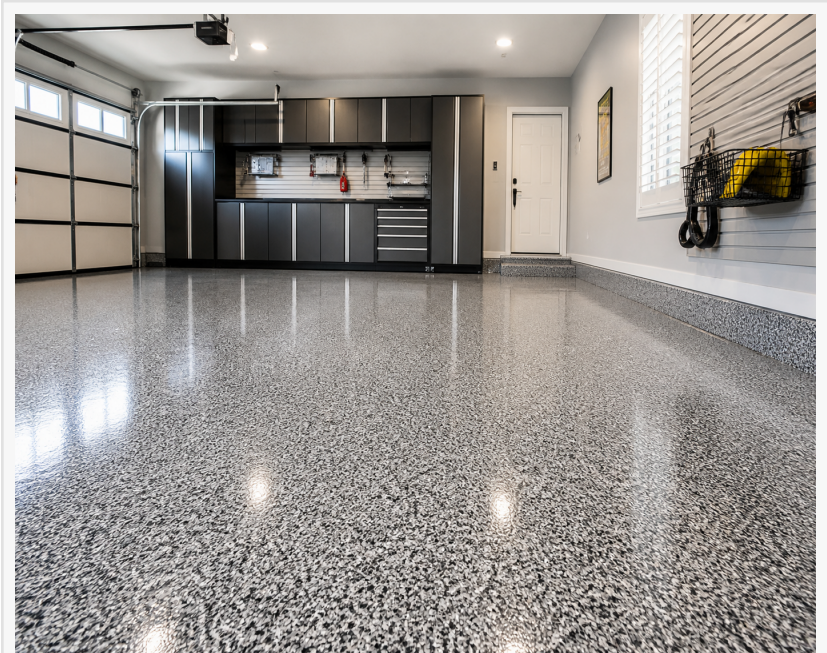
Professionally installed epoxy flake garage floor coating in Queen Creek, AZ — diamond ground, crack repaired, and coated in a single day.
