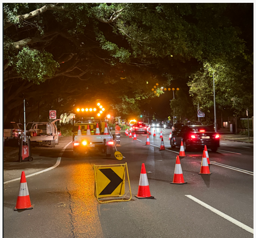
Traffic Management Company Sydney performing night shift roadworks.
