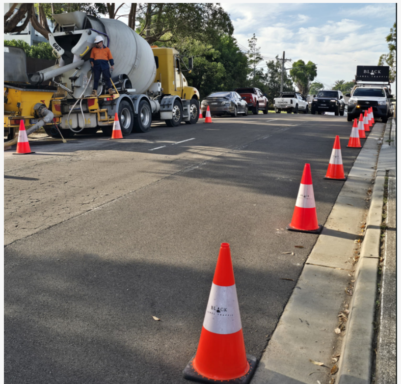
Traffic Control for concrete pours
