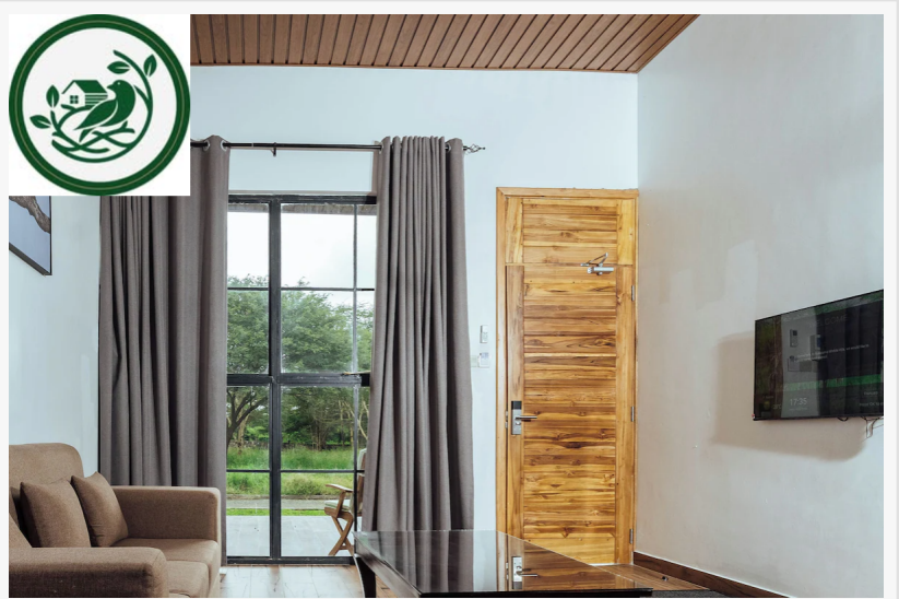
A photograph taken inside a room at the Aya Sophia Wildlife Resort, featuring installed FMUSER IPTV and a smart door lock.
