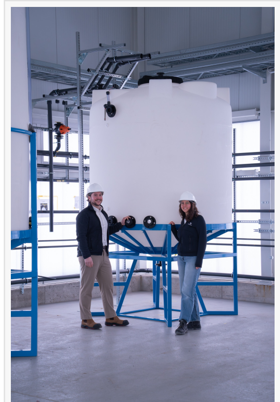
Inside our Industrial Plant
