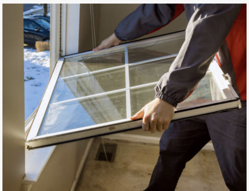
Window Solutions Window Installation
