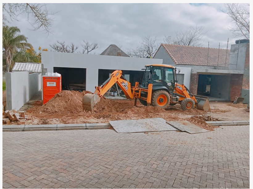
paving in cape town
