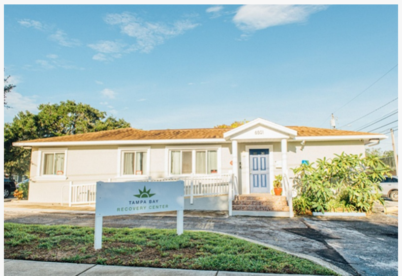
rehab in Tampa
