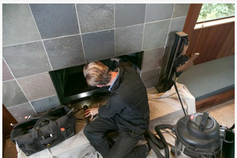
fireplace repair service in Mill City OR..
