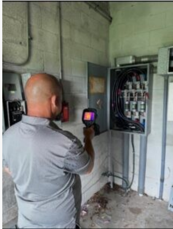
infrared thermography inspections
