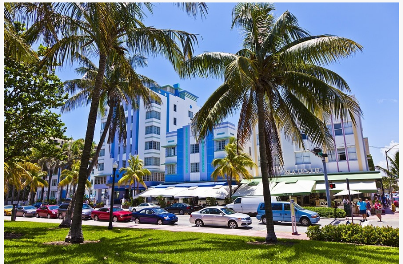
Miami-Dade 40-Year Building Recertification inspection services
