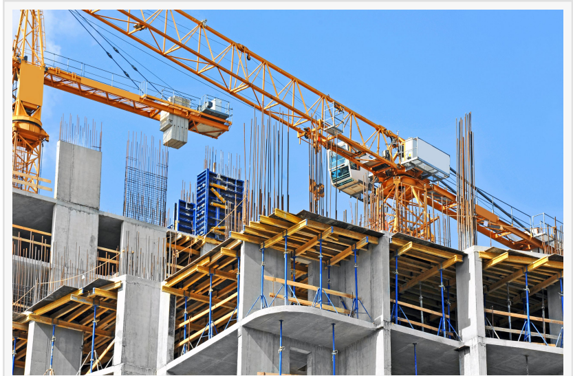
Construction Site Work
