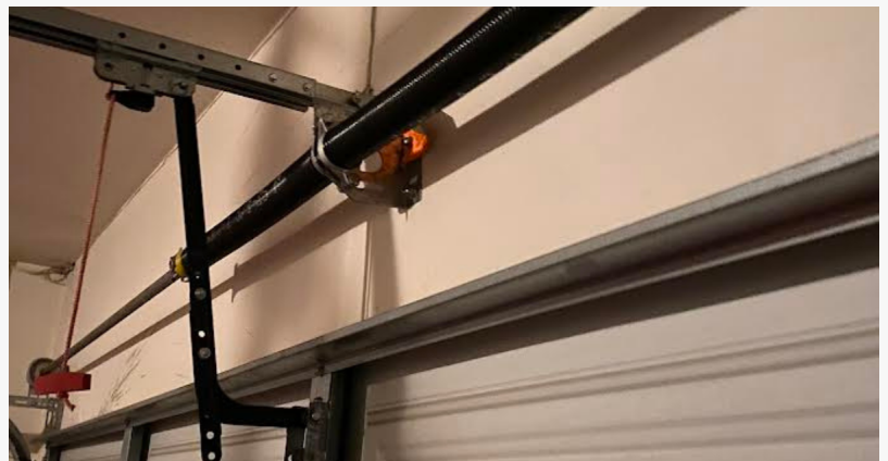
24/7 emergency garage door repair service in Pasadena
