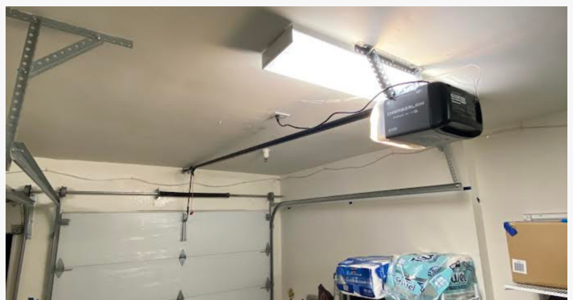
Emergency broken garage door spring replacement in Pasadena
