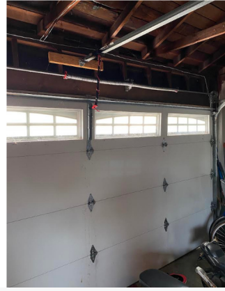
Off-track garage door repair near Pasadena neighborhoods
