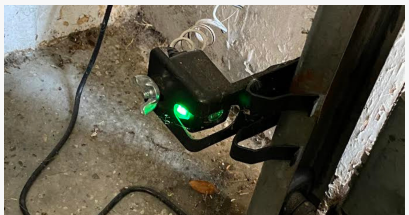
Same-day garage door repair service in Pasadena CA
