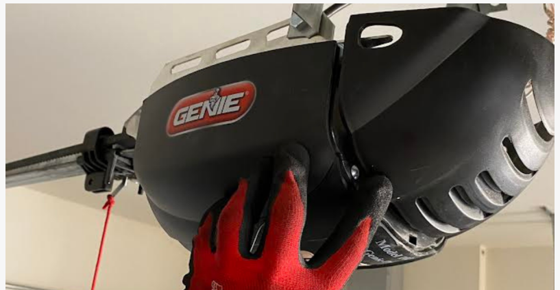
Garage door opener repair for Pasadena homeowners
