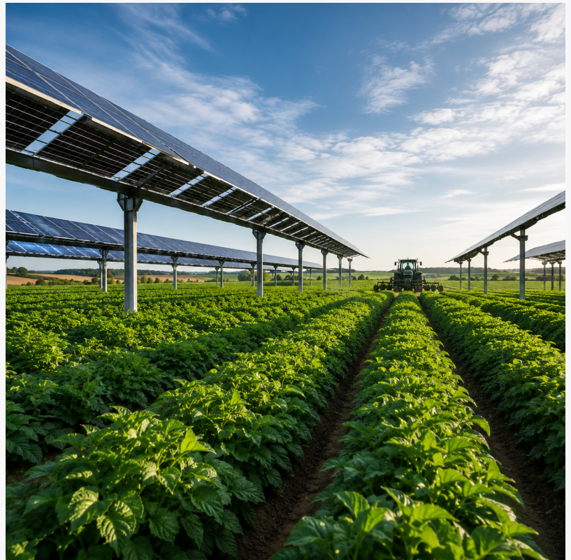
EnergyLane's agrivoltaic system
