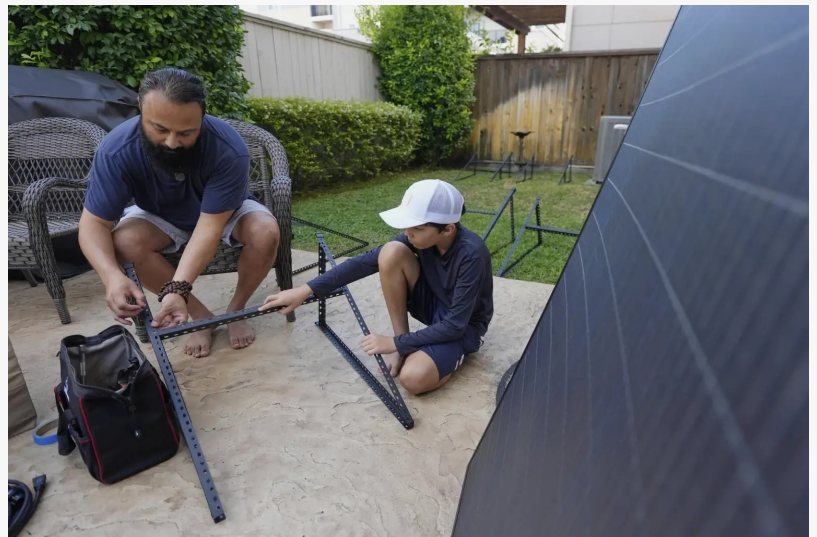
Installing CraftStrom solar kits is easy and can be a household project.
