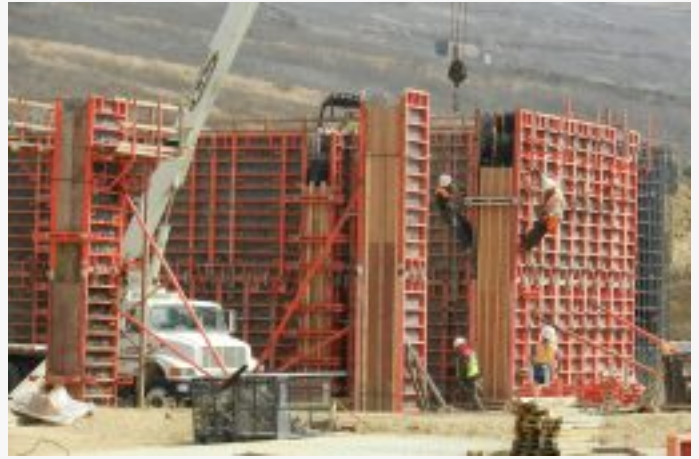
R. Dugan Construction, Inc. completed work on the Olinda Landfill Gas to Energy project in Brea, California, one of the company's largest completed projects.
