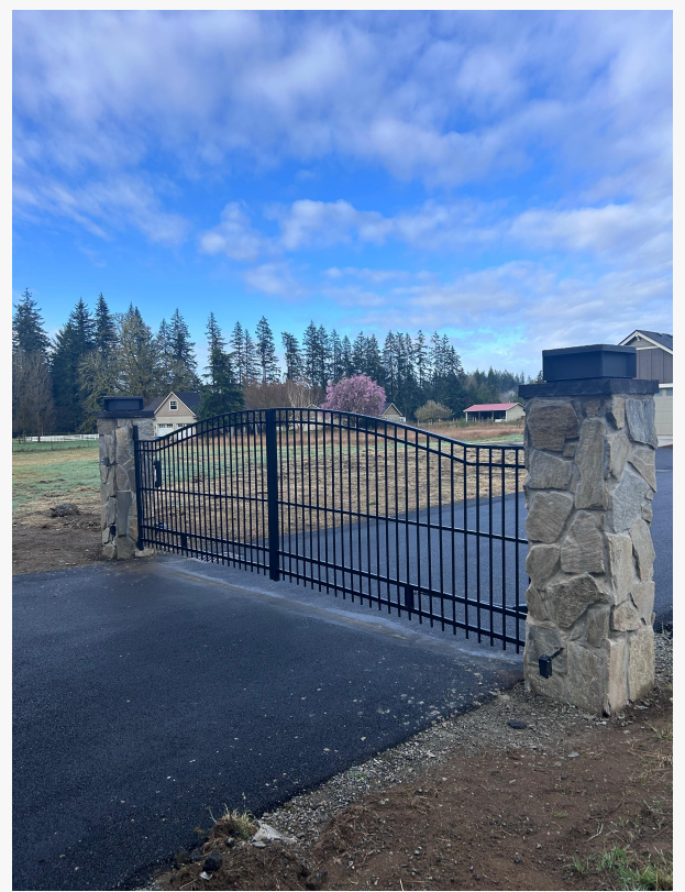
Stone pillars with Driveway automatic gate fully custom in WA
