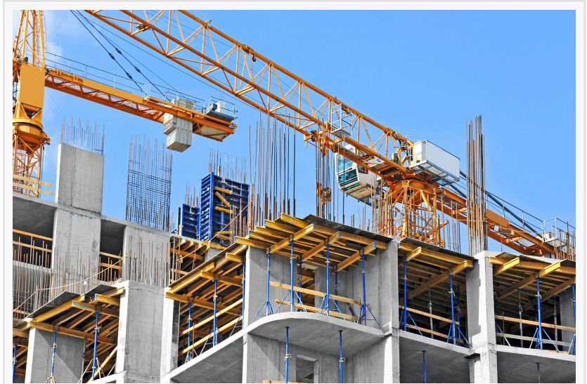
Construction Site Work
